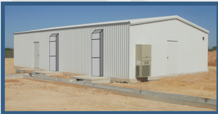
Pulling Vaults w/ Aluminum Risers (Beside Control House)
