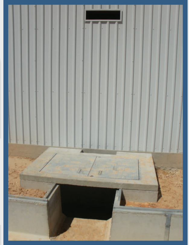
Pulling Vault (Building End)
