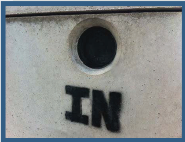
Pipe Seal Openings
